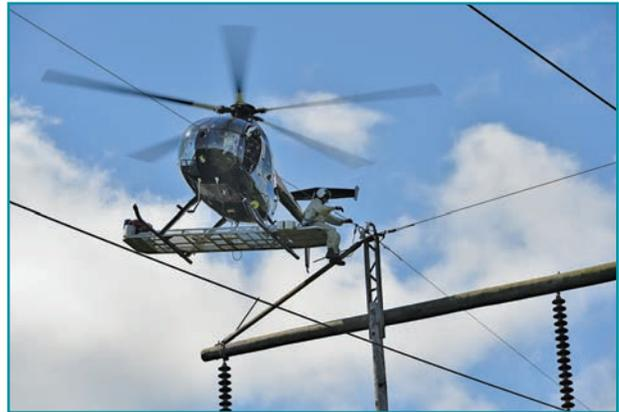
**figure 2.** An aerial installation of optical ground wire. (Source: NYPA; used with permission.)
